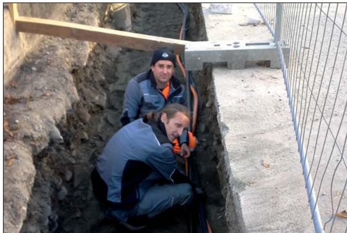
Breitband-Baustelle in Alt-Debant
